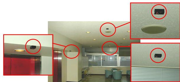
Figure 3. An example of arranging IrDA markers.
